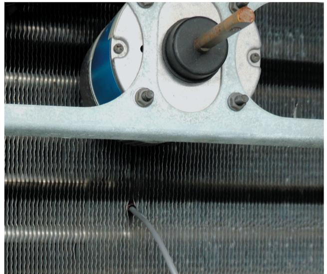
3a. Connect the Evaporator Coil Ice Sensor to terminals ICE1 & GND per the wiring diagram on Page 7.
